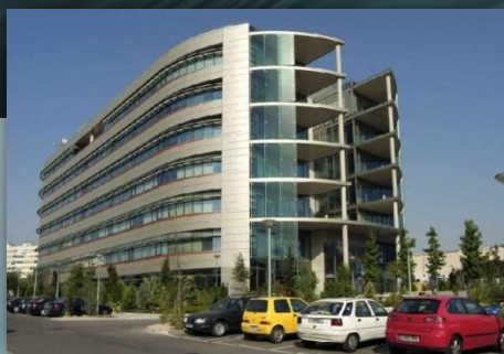
Alvento - Metrovacesa Business Park (Madrid)
